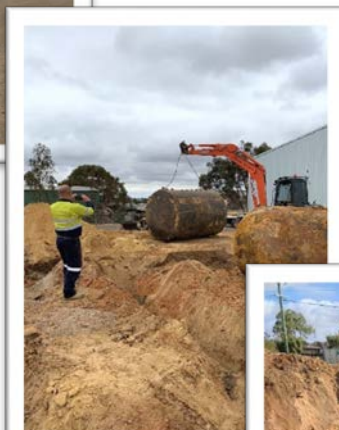
Removing the tanks
