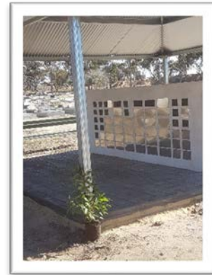
Niche wall after
