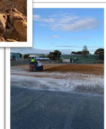
Depot yard after the tanks have been removed
