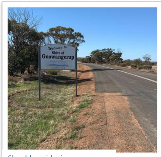
Shoulder widening Gnowangerup - Tambellup Rd
