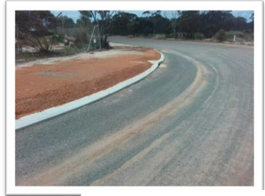
Kerbing and sealing on the corner of Quinn and House St
