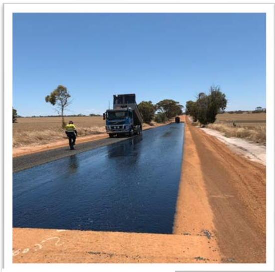
Sealing Kwobrup Road
