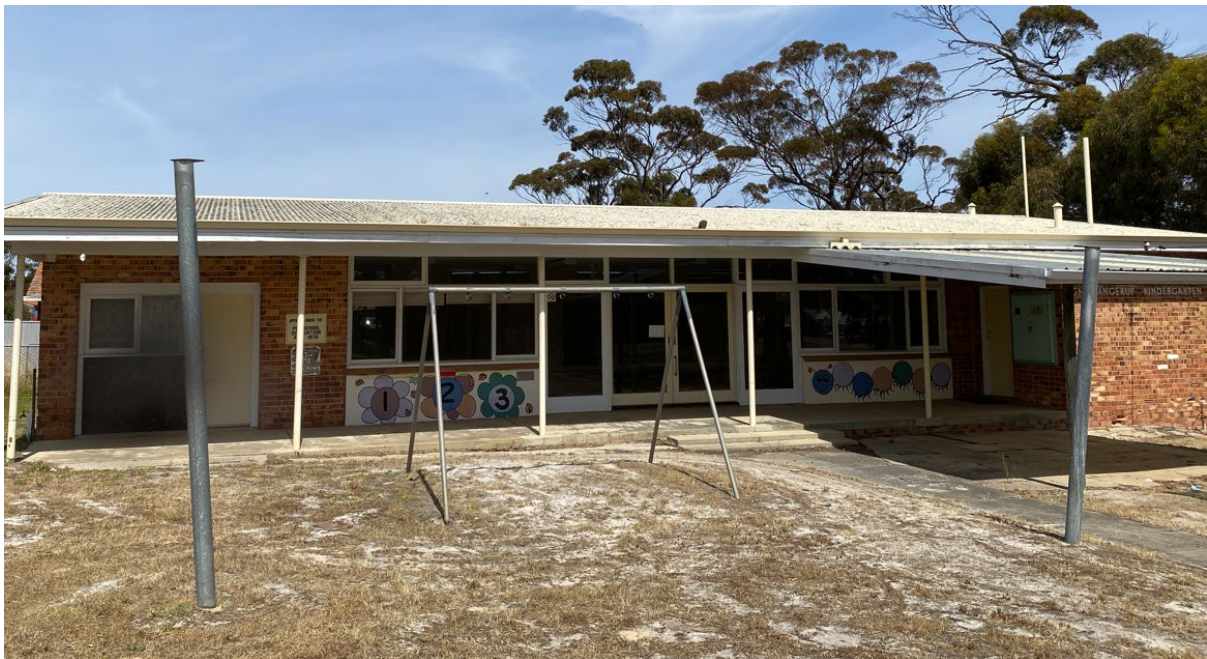
Figure 4: Old Kindergarten Building situated at Lot 418 Whitehead Rd
